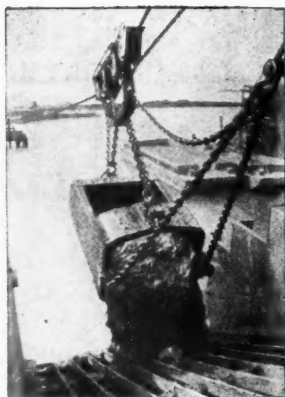
This Sauerman Bucket Lifts 5 Tons of Material Per Trip; Makes 60 Trips An Hour.
